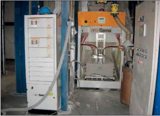
Figure 5. ITW Gema electrostatic spray control system used on the vertical powder line.
